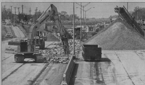
Broken concrete from the demolition of I-96 will be ground into gravel for the reconstruction. BILL BRESLER / STAFF PHOTOGRAPHER
