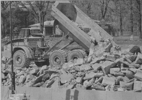
Broken concrete, piled high, will be ground into gravel for the reconstruction.
