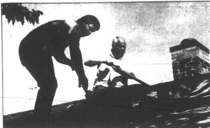
Dan and Carson Coonce rip off the old roofing.
