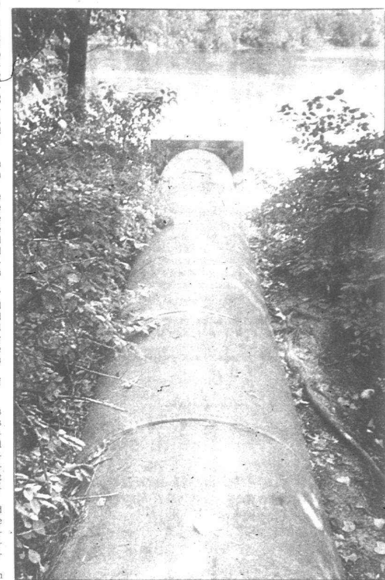
Some 180 combined sewer overflows (CSOs) were built instead of separated storm drains and sanitary sewers. When they overflow, they pour six billion gallons of wastes annually into the Rouge, making it "the dirtiest river in Michigan."
