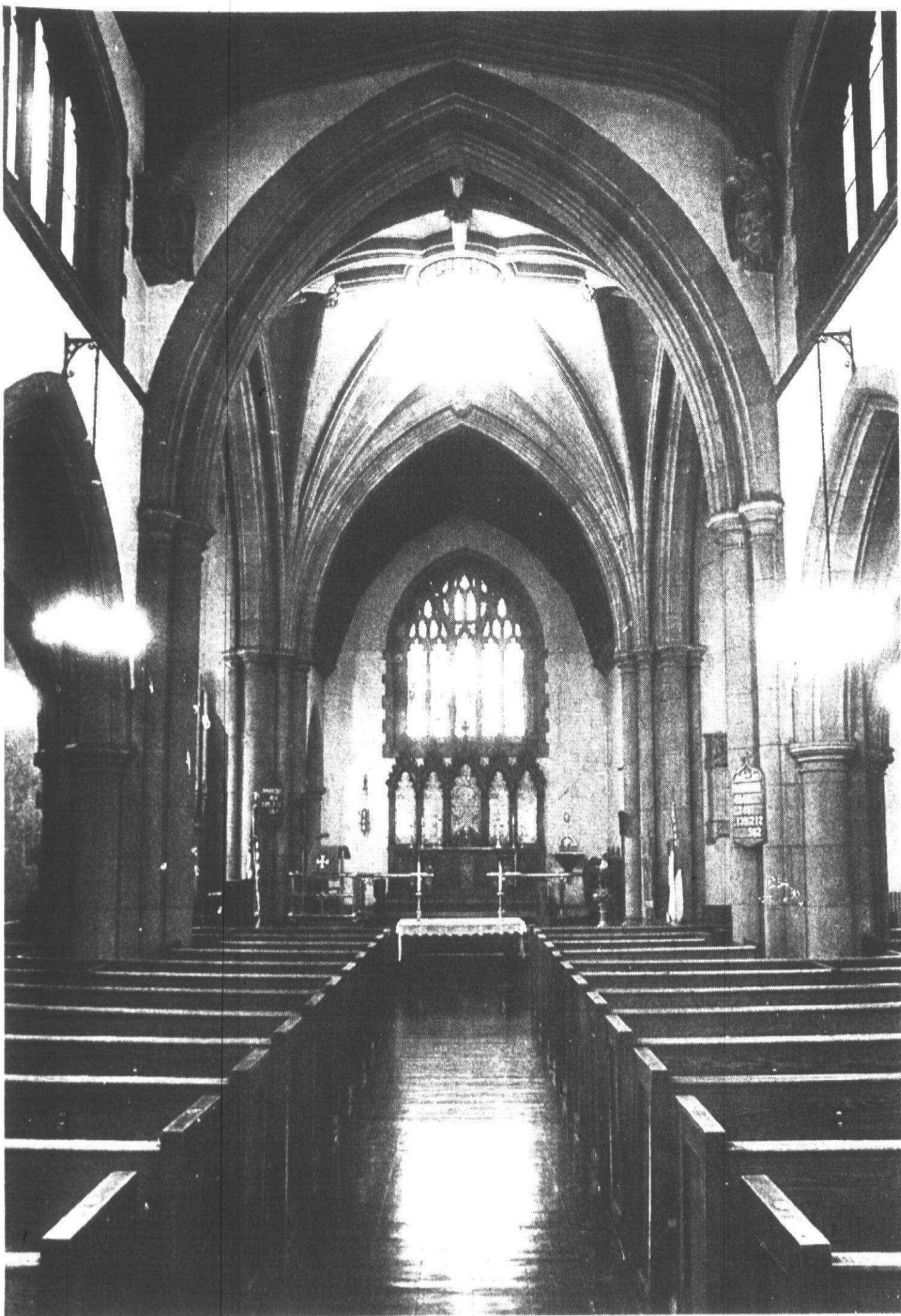
Trinity Episcopal, built in 1893, is constructed entirely of stone with a small amount of wood. The outer walls are two feet thick.
