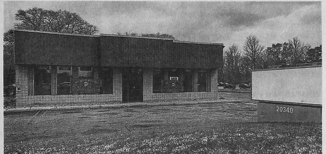
The former Napa Auto Parts store on Farmington Road in Livonia could be demolished to make way for a new car wash. DAVID VESELENAK/HOMETOWNLIFE.COM
