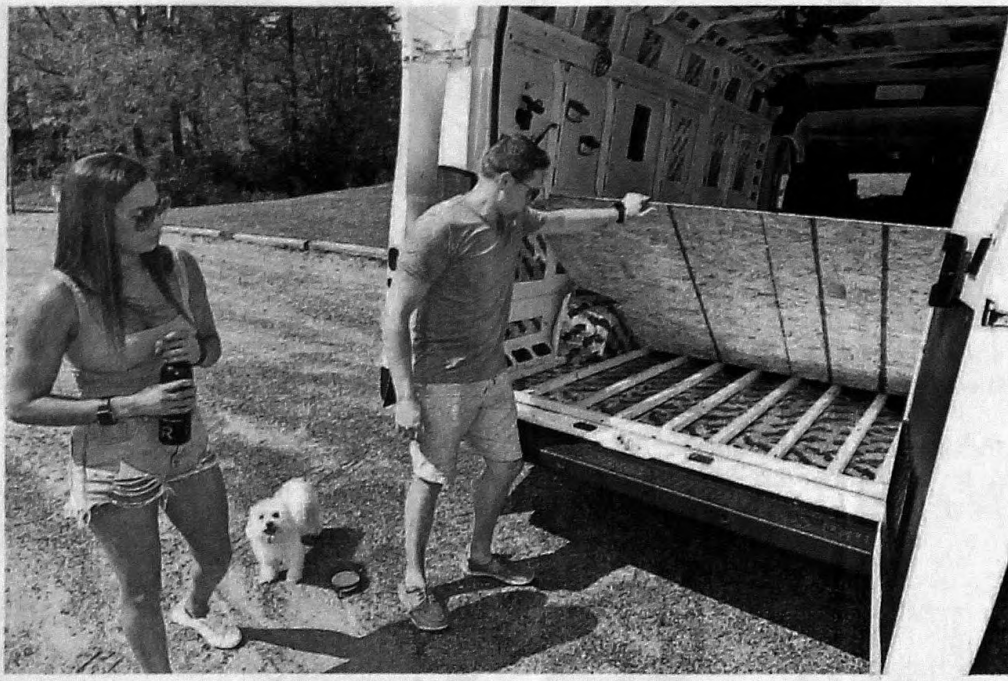
In this summer of 2021 image Erica Battle and Nick Kokenos show off how they're placing particle board under and around their Ram ProMaster conversion van to place insulation in it to keep them cool in the summer and warm in the winter.
