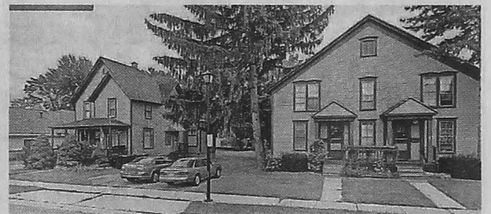
Two of the three structures that were demolished the week before Christmas. COURTESY OF GOOGLE MAPS
