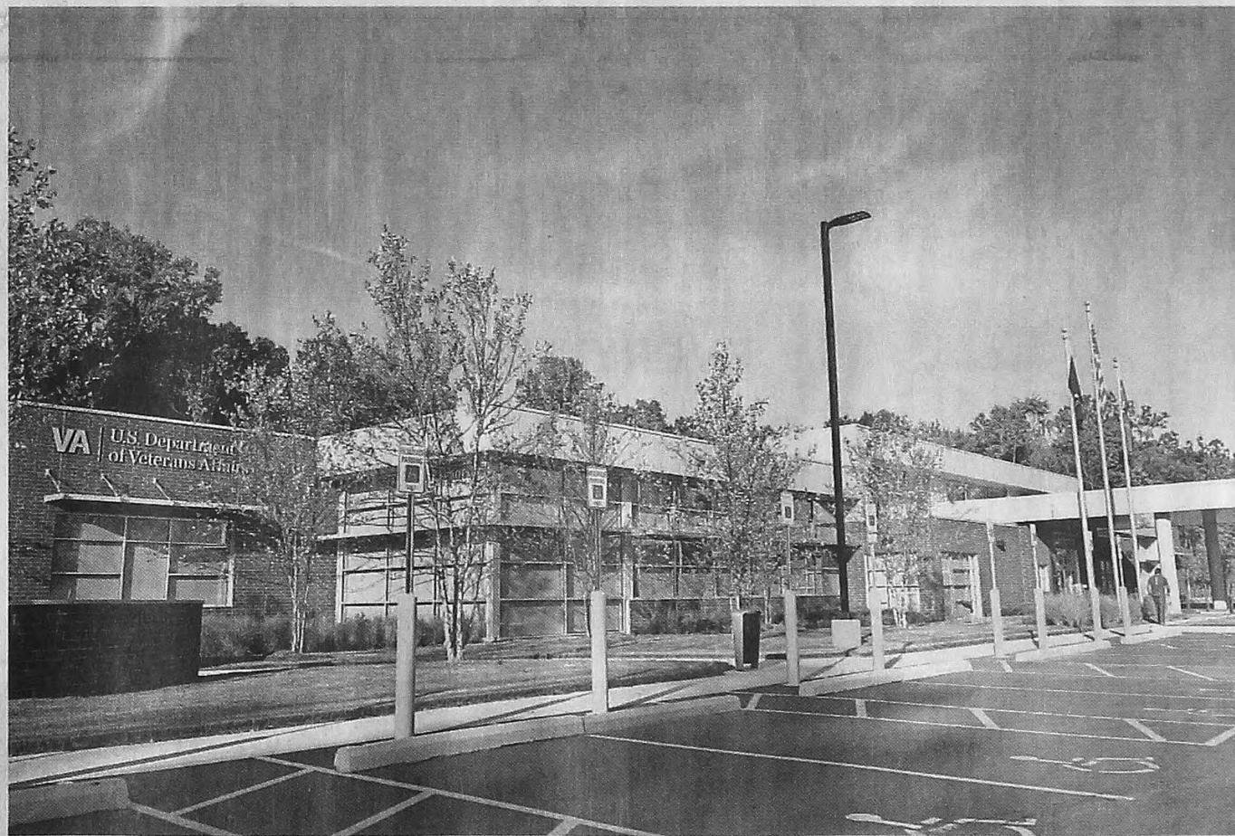
The new U.S. Department of Veterans Affairs Canton Community Based Outpatient Clinic on North Lotz Road is nearly complete. JOHN HEIDER/HOMETOWNLIFE.COM
