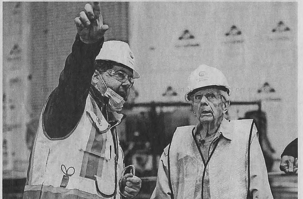
Michigan Central construction manager Richard Bardelli, left, guides Joe England for a tour inside of the Michigan Central Station in Detroit on Sept. 25, 2021. JUNFU HAN, DETROIT FREE PRESS
