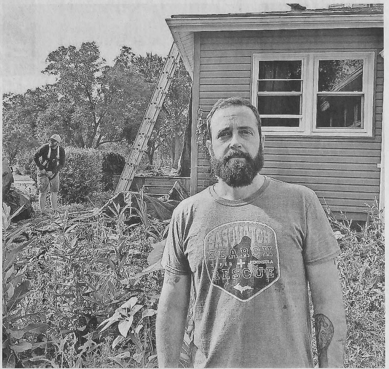
Canton resident and Army veteran Carson Middlebrook was beyond appreciative of his home's new roof.
