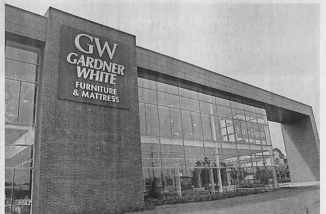
New signage adorns the building along Ford Road that used to hold Art Van Furniture and Love's Furniture & Mattresses.
