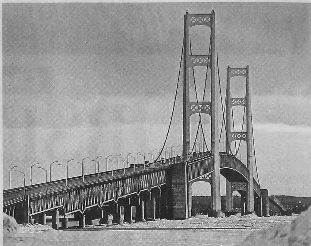
Traffic moving along the Mackinac Bridge seen from the Upper Peninsula.
