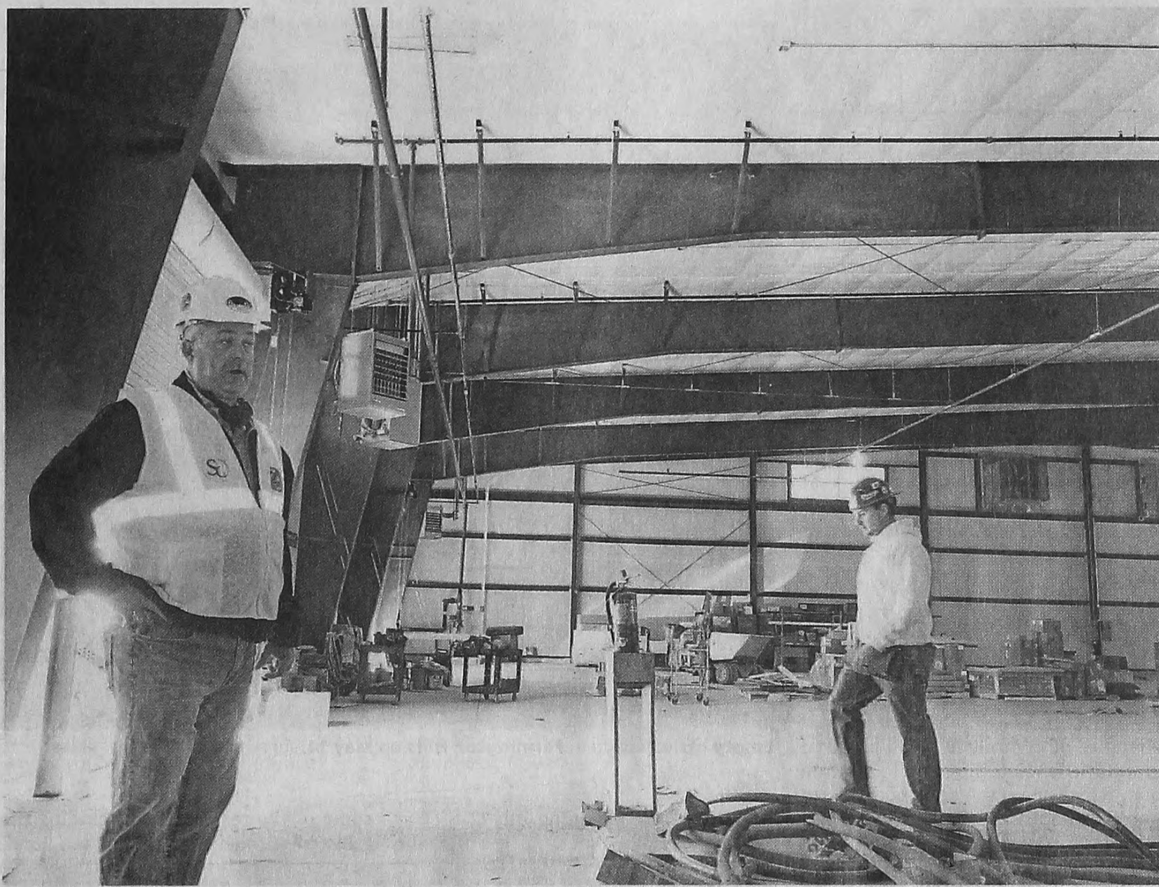
Director of Public Service for Livonia Donald Rohraff, left, stands inside the city's new DPW building May 12. The garage alone, with no support posts getting in the way of the large vehicles that will use it, takes up 21,000 square feet.
