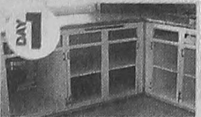
Existing cabinets are prepared for the refacing process
