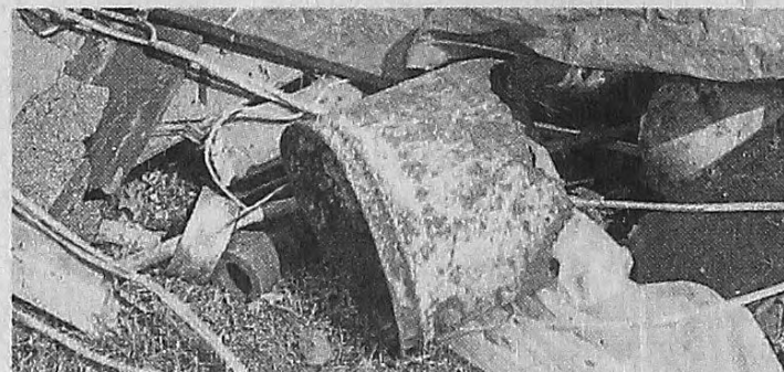
The crew set aside metal and pipes for recycling.
