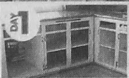
Existing cabinets are prepared for the refacing process.
