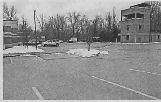
Novi's Fire Station No. 4 at 49375 Ten Mile Road, with ample parking at its site, is slated to be used as a COVID-19 vaccination center in the future.
