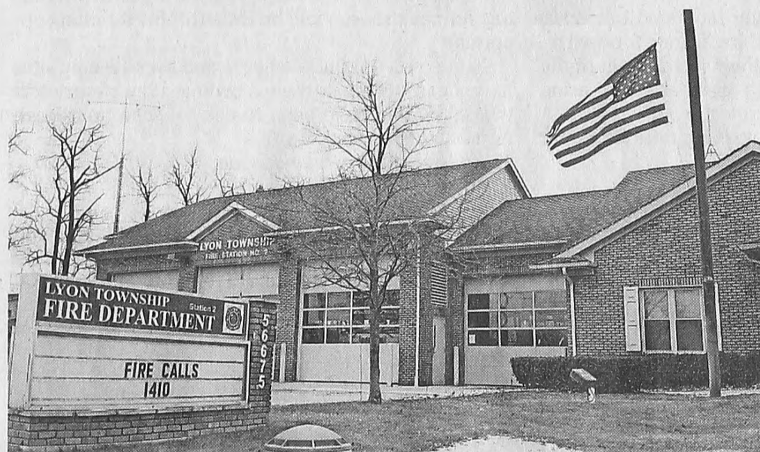
Lyon Township’s Fire Station No. 2 sits along Ten Mile Road near Milford Road. JOHN HEIDER/HOMETOWNLIFE.COM
