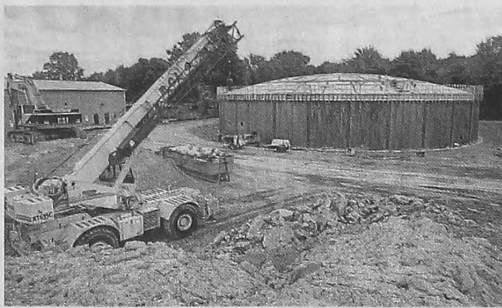
Canton Township built a 2.5-million-gallon water storage facility near Joy and Morton Taylor in 2016 to help manage water rates for residents and businesses in the township. HOMETOWNLIFE.COM FILE
