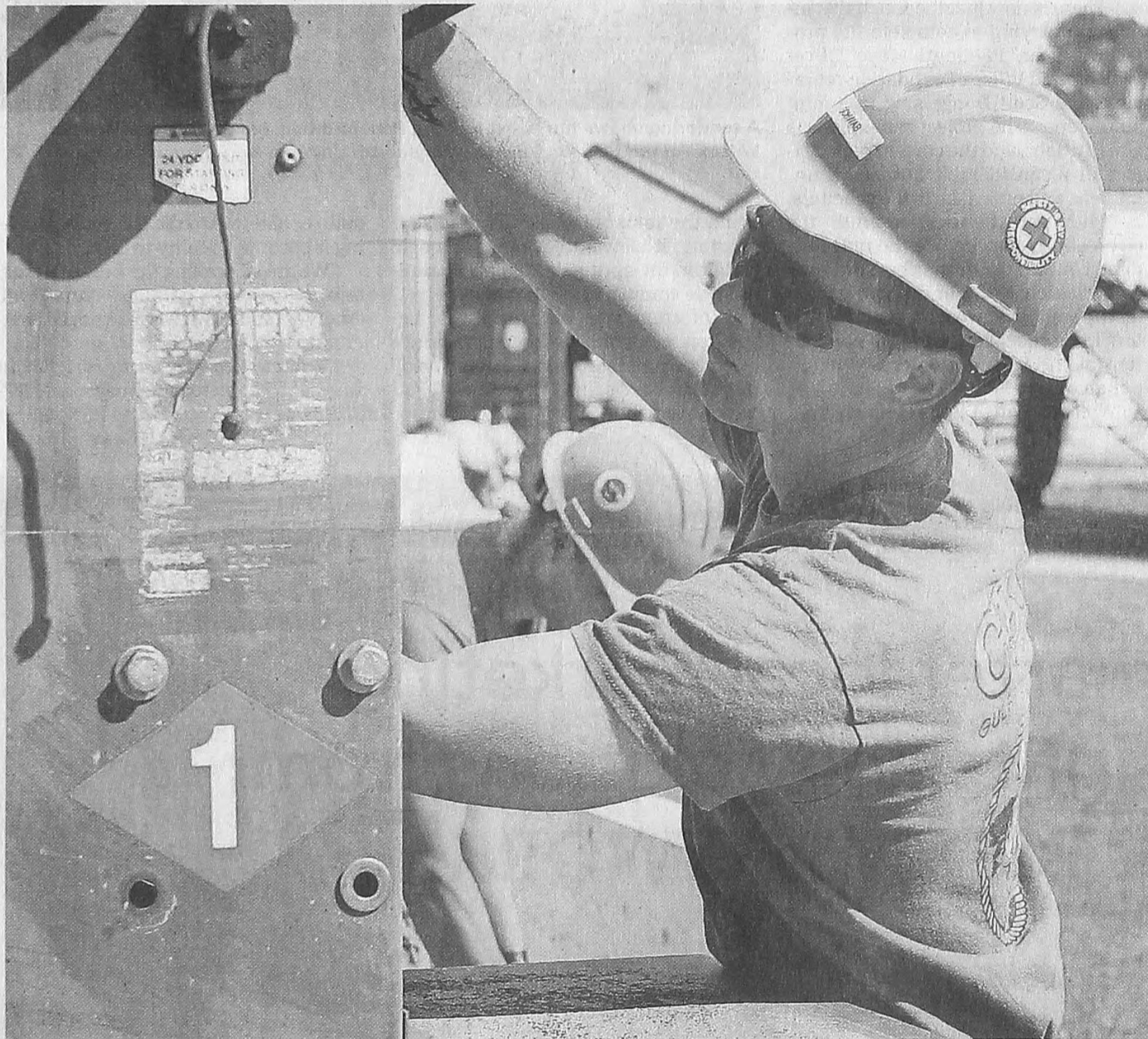
Builder Constructionman Steven Schwab, of Westland, assigned to Naval Mobile Construction Battalion 1, inspects a lighting unit for a pre-staging area in front of Naval Hospital Rota in southern Spain. PHOTOS COURTESY OF CAINE STORINO
