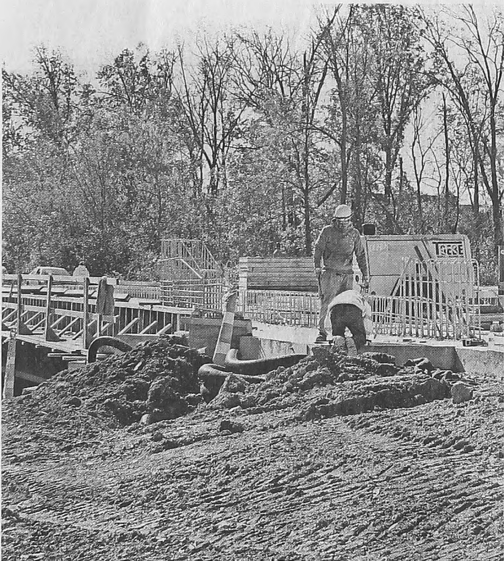
Work continues Oct. 23 on the replacement of a bridge on Lilley Road just north of Michigan Avenue in Canton Township. JOHN HEIDER/HOMETOWNLIFE.COM
