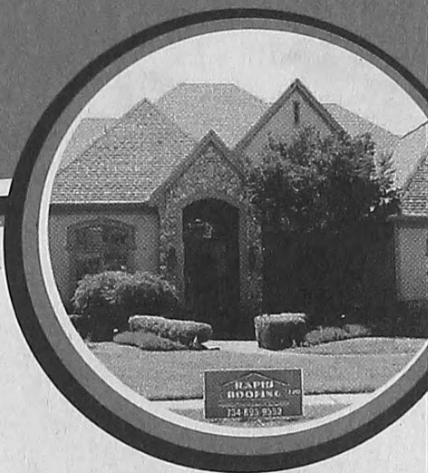
Actual Rapid Roofing Completed Project
