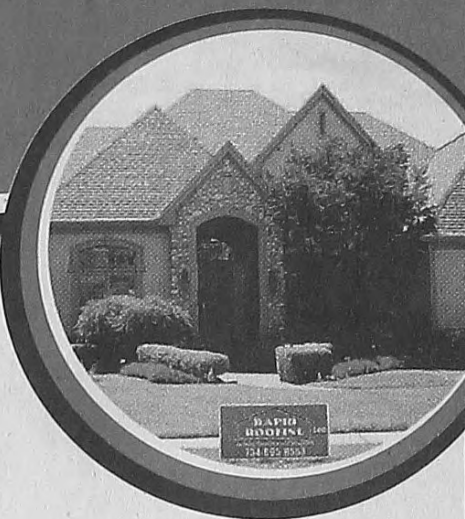
Actual Rapid Roofing Completed Project
