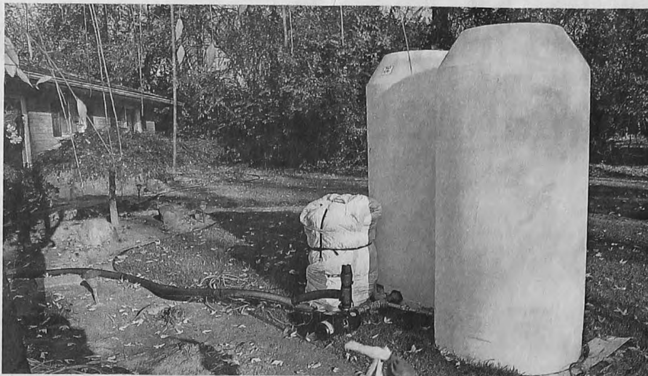
Two water tanks outside of resident Justin Droste's house.
