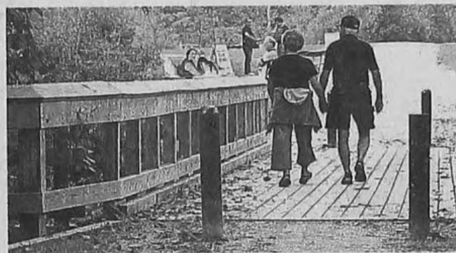
FILE PHOTO Bridge work has been completed on the Lower Rouge River Recreation Trail.
