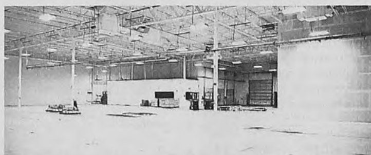
This 53,000-square-foot facility in Novi will house Google's self-driving vehicle development center, the company announced Wednesday.
