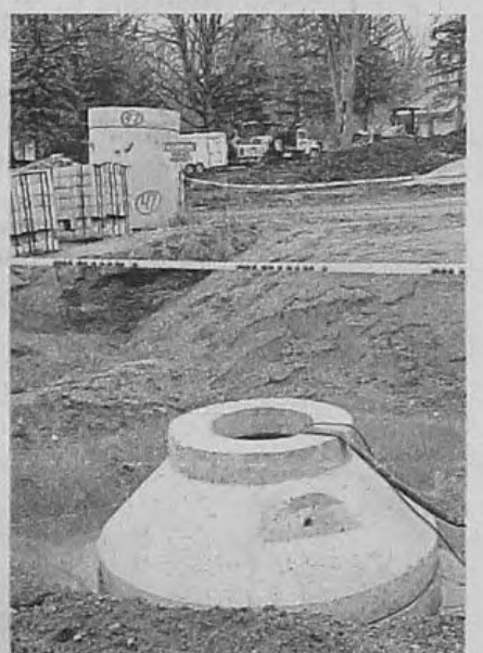
BILL BRESLER | STAFF PHOTOGRAPHER Lotz Road's infrastructure is being improved.
