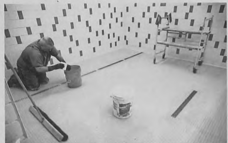
New tile is being installed in the men's locker room.
