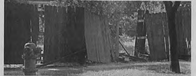
BILL BRESLER | STAFF PHOTOGRAPHER Noreen Armstrong's privacy fence was damaged recently by a car.
