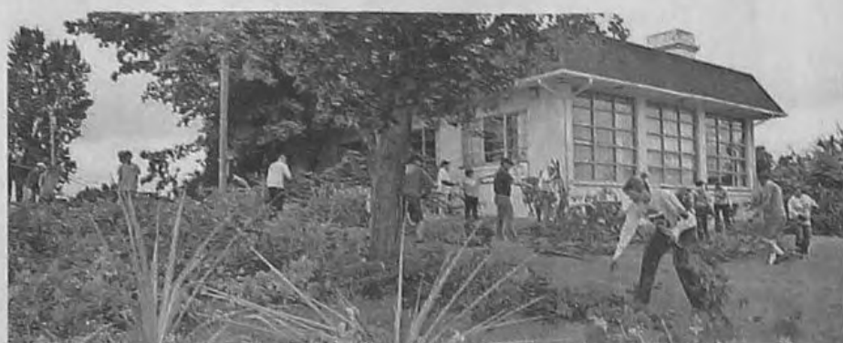
The site, near Cherry Hill and Ridge, is being transformed into the Village Arts Factory.
