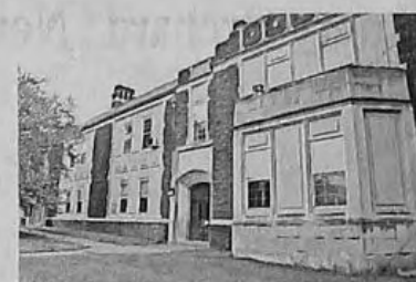
BILL BRESLER | STAFF PHOTOGRAPHER The former Starkweather School is at the center of an effort to preserve Plymouth history.
