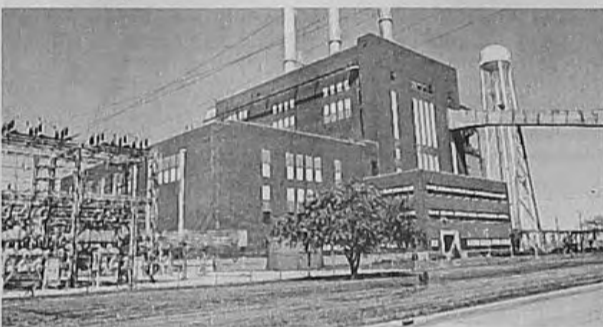
Consumer's Energy J.R. Whiting Generating Complex on an 875-acre site along the Lake Erie shoreline in Erie is one of the smallest coal-fired plants in the company's fleet. It began producing electricity in 1952.
