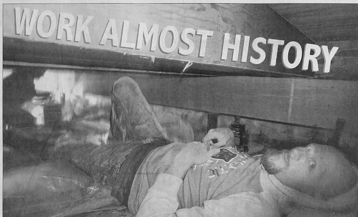
Rob Oliver works under the museum in a claustrophobe's nightmare of a space that is less than three feet deep. Standing water had to be pumped out and a drainage system installed to keep the crawlspace dry. Floor joists were reinforced and replaced. The stone foundation was repaired. He and the rest of the crew work for D&P Caulking and Restoration. PHOTOS BY BILL BRESLER | STAFF PHOTOGRAPHER
