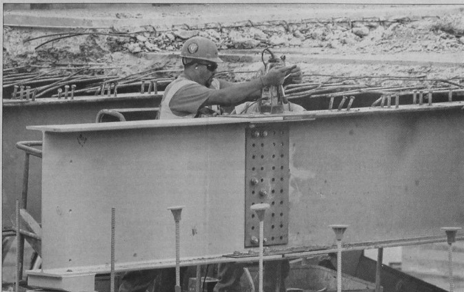
A construction worker installs new fasteners designed by Livonia-based AlphaUSA on the Melvin Street bridge as a part of the I-96 reconstruction project. The bridge was the first place in Michigan where AlphaUSA's new product was installed.
