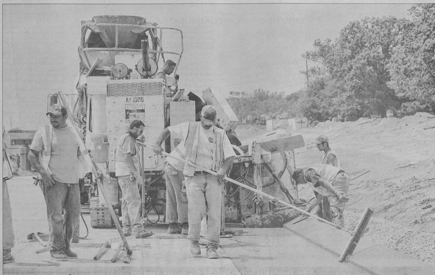
The concrete shoulder is formed and finished. PHOTOS BY BILL BRESLER | STAFF PHOTOGRAPHER
