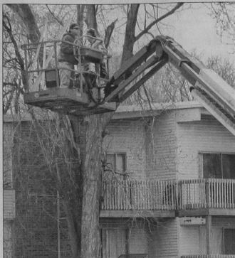
Maintenance crews could be seen working Thursday afternoon at The Crossings at Canton. BILL BRESLER | STAFF PHOTOGRAPHER
