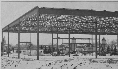
Construction has begun on the new La-Z-Boy store in Canton, on Ford Road west of Lily. BILL BRESLER/STAFF PHOTOGRAPHER
