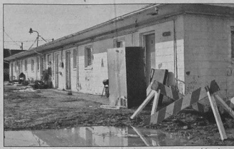
This small apartment building, condemned by Canton Township, sits off of the eastbound lanes of Michigan Avenue at Morton Taylor. BRESLER / STAFF PHOTOGRAPHER
