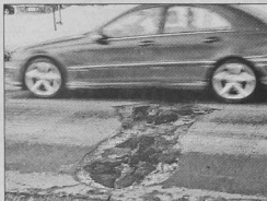
There are far too many massive potholes in Michigan. JOHN STORMZAND/STAFF PHOTOGRAPHER
