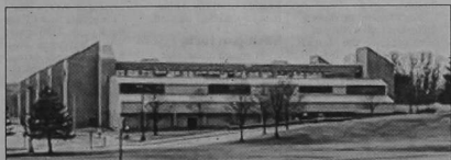
Harrison High School was evacuated Friday evening after a small fire developed in an electrical room. No injuries were reported.
