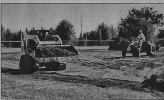
Workers were busy this week repairing baseball fields at Griffin Park. GREATER CANTON YOUTH BASEBALL SOFTBALL ASSOCIATION
