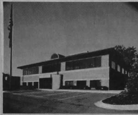
The D. J. Maltese Building Dearborn
