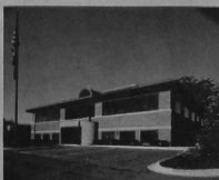
The D.J. Maltese Building Hudson
