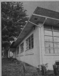
The factory and offices at the southwest corner of Cherry Hill and Ridge were commissioned by Henry Ford. BILL BRESLER | STAFF PHOTOGRAPHER
