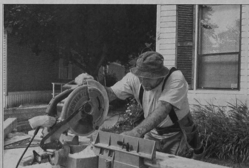
Pat Lindstrom of South Lyon cuts a top board for Chuck Langham's new deck.
