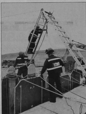
Stabilizing the trench walls and building the tower that supports the Vector hose.
