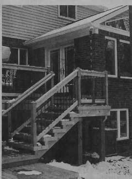
"Upstairs Downstairs" two-story addition and deck by Seghi Renovations.
