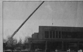
Workers installed a new emergency sign last week in preparation for Wednesday's opening of the new Emergency Center at St. Mary Mercy Hospital, Livonia.
