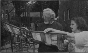
The Rutherfords fit the stained glass panels into the metal-work earlier this month.
