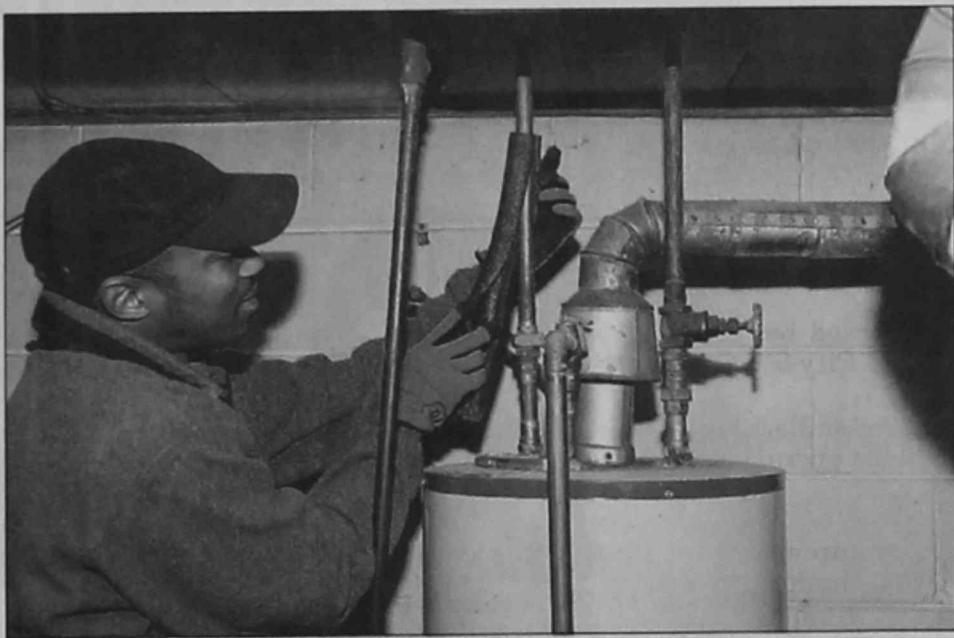
As part of DTE's home energy consultation program, energy consultants will install wrap on the water heater pipes — up to nine feet from the hot water tank — an energy-saving measure that can reduce heat loss and increase water temperature in the pipes.
