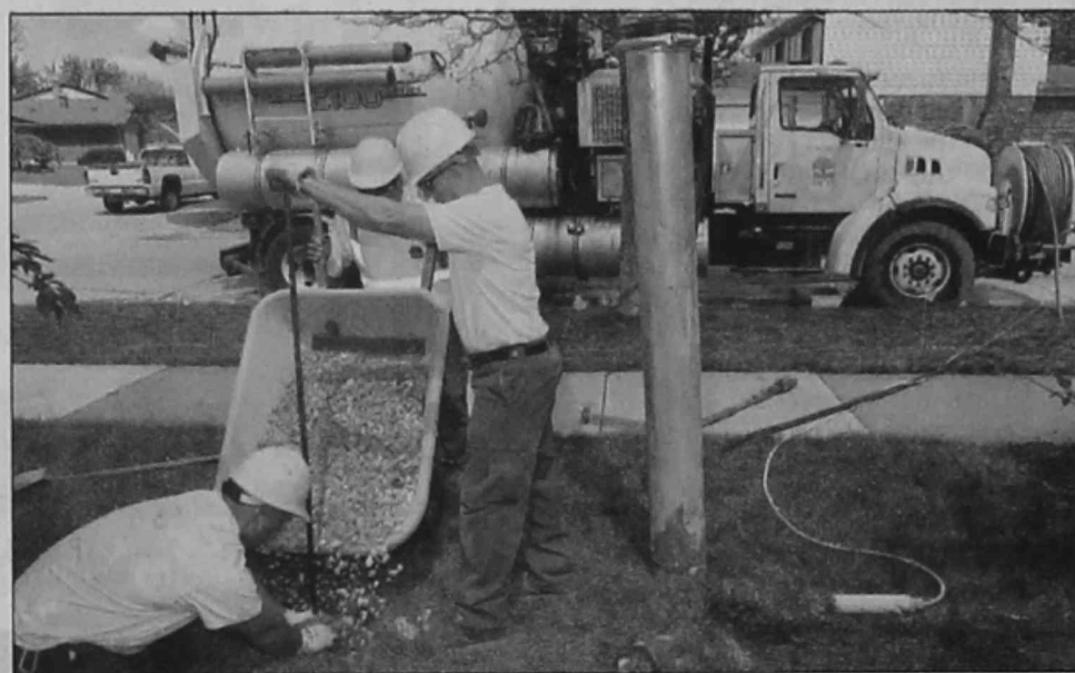
John Fox, Craig Cromie and Jay Herdon finish repairing a water shutoff valve in a Canton neighborhood.
