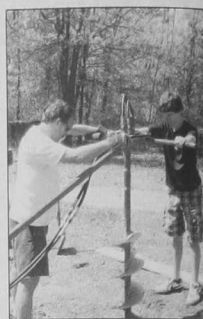
Cody Murphy and his father Jerry use a gas-powered auger to drill holes to cement in the posts for benches erected at the library pavilion.
